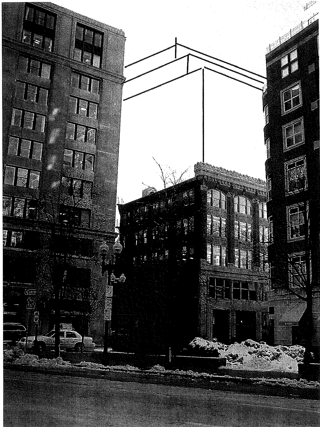
4. From Park Plaza Hotel Entrance
