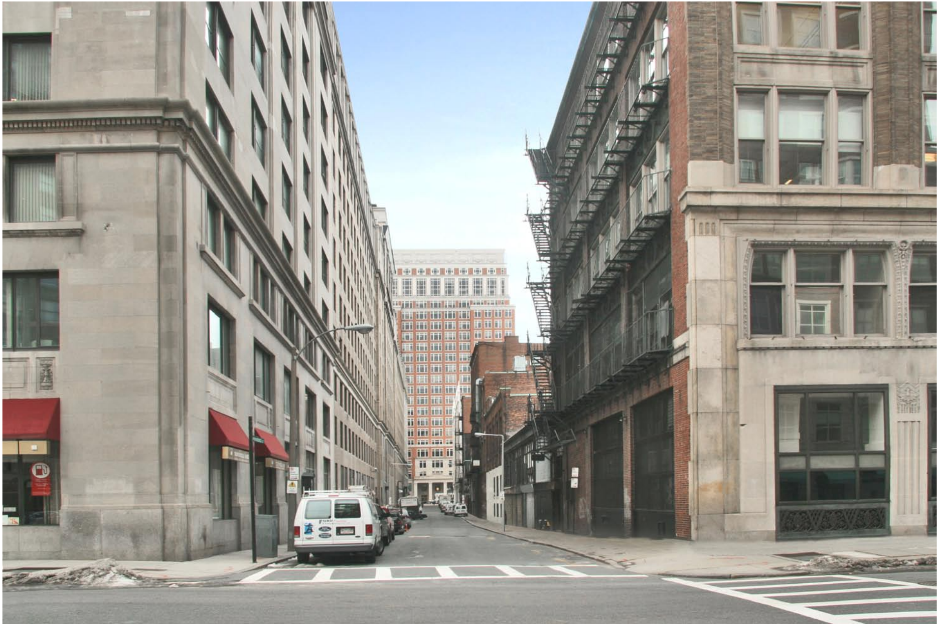
Current Providence Street View Looking West
