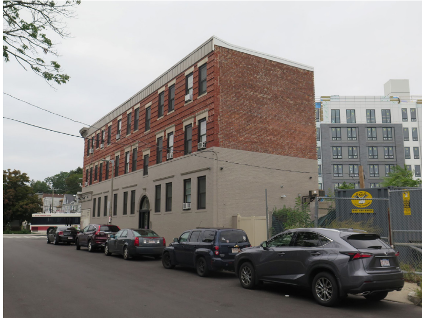
Ashmont Landing Apartments at the Corner of Beale Street and Dorchester Ave
