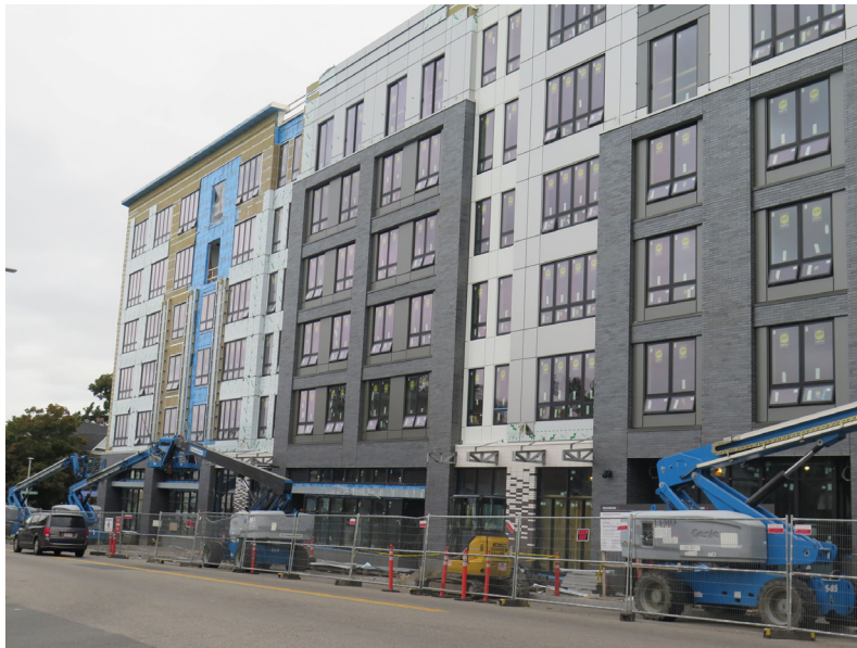
Mixed-Use 1975 Dorchester Ave Building Under Construction Across from Site
