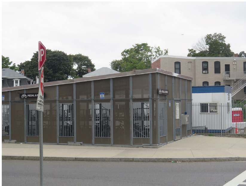
Existing MBTA Bike Storage Building Adjacent to Site
