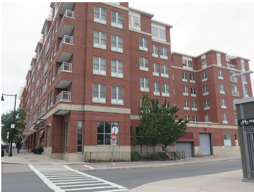
Existing Building Along MBTA Access Road Near the Site
