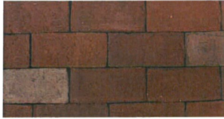
Brick Paving In Frontage Zone
