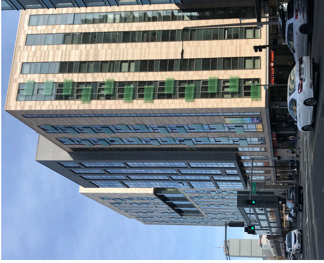
12. Boylston Street, Boston, MA. Looking Southeast.
