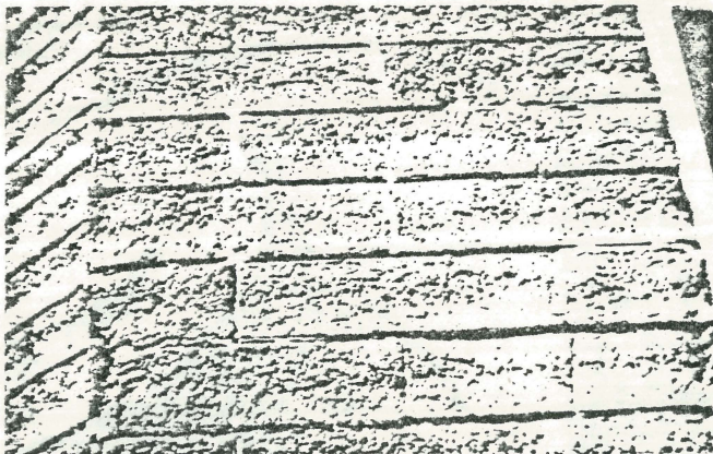
Figure 5. This brickwork was sandblasted to remove paint. Note the severe erosion which has occurred, especially in the softer center sections of this "hard burned" late 19th-century brick. Although this is a severe example, the same problem of increased roughness and porosity will occur even on more skillfully performed jobs where the effect is less evident visually.
