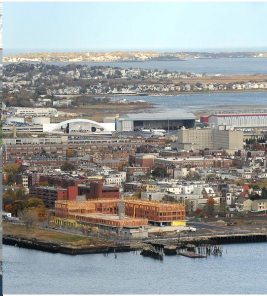
Pier 1, East Boston
