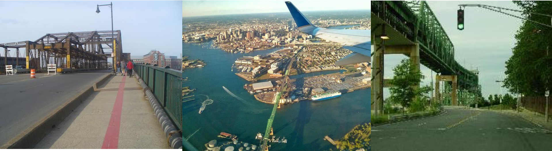
Bridge Infrastructure (North Washington Street Bridge, Tobin Bridge)
