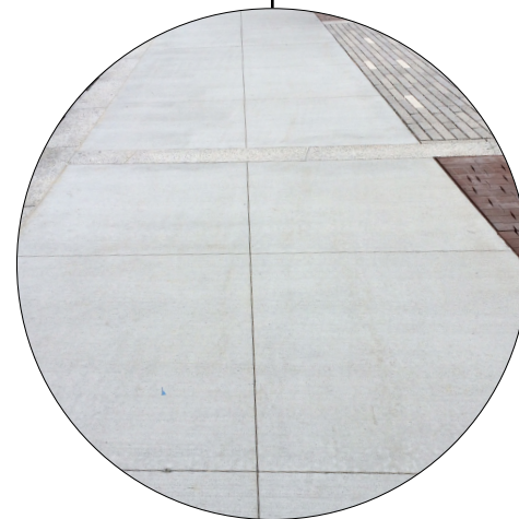
CONCRETE WALKWAY WITH SAWCUT JOINTS
