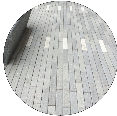
PERMEABLE PAVING
