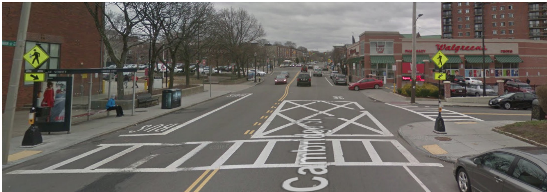
Pedestrian improvements on Cambridge Street near Union Square included accessible curb ramps, pedestrian crossing signs, and enhanced pavement markings.
