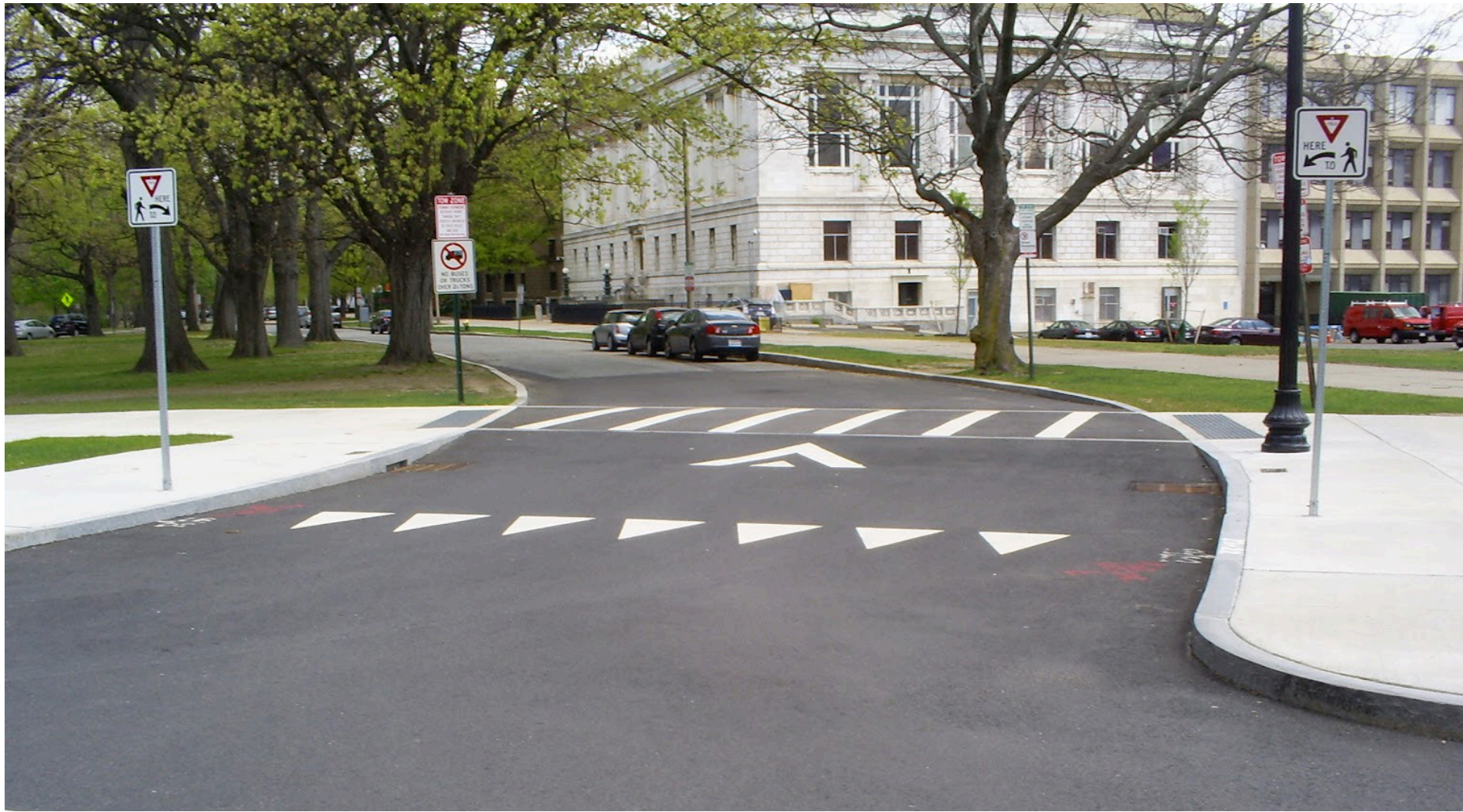
A raised crosswalk in Boston’s Fenway neighborhood ensures safe pedestrian crossings and slows traffic.
