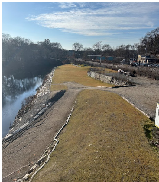
Former Lewis Chemical site
