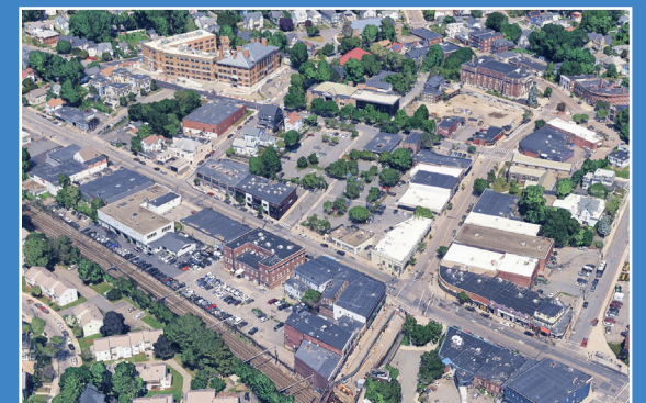
Aerial photo of the municipal parking lot
