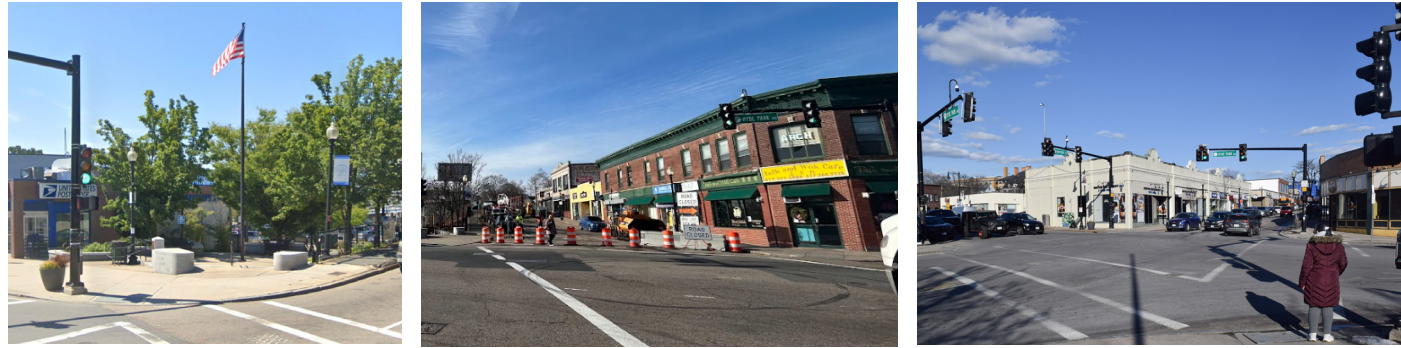
Pocket Park, Hyde Park Ave and River St The Fallon Building, Hyde Park Ave and River St Storefronts, Hyde Park Ave and River St
