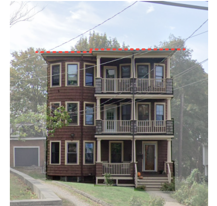
Example of a flat roof
