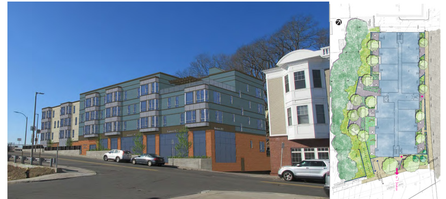
Article 80 approved project Imagery - Full approved project can be found on line on: https://bpda.box.com/s/3zurh76afxberjrtiyi305nfy24h7r2
