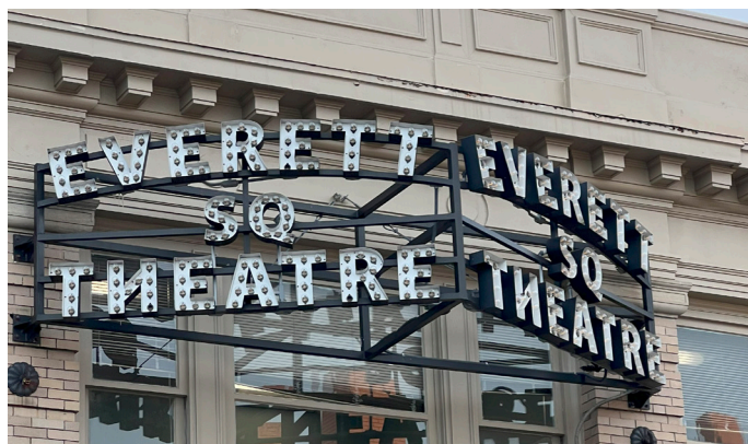
The Everett Square Theatre restored marquee
