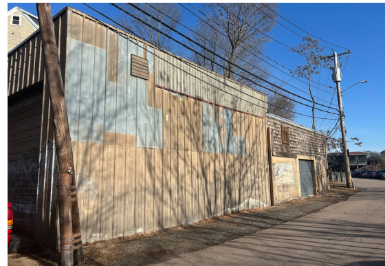
Garage on Walnut St
