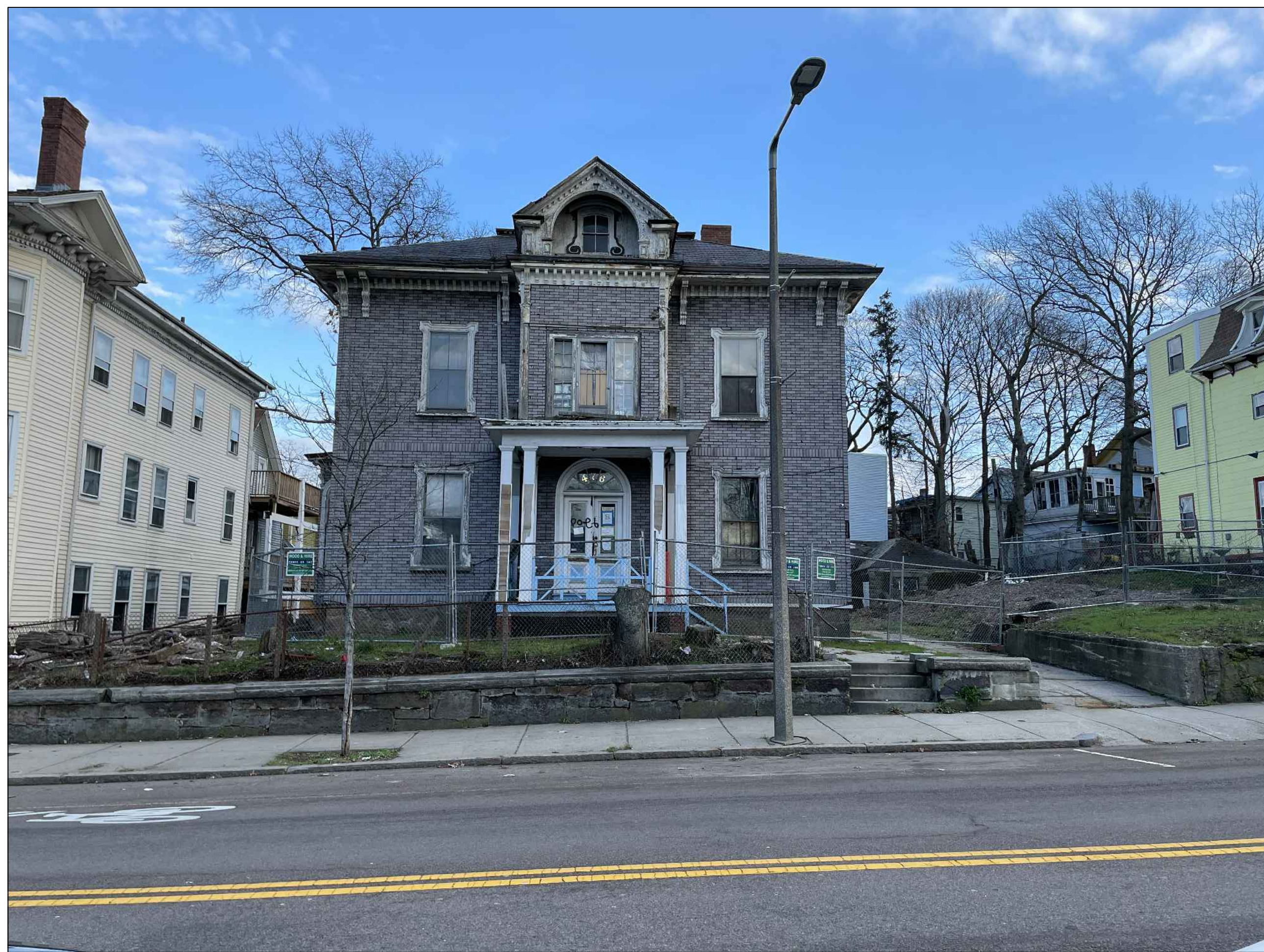
FRONT FACADE EXISTING
