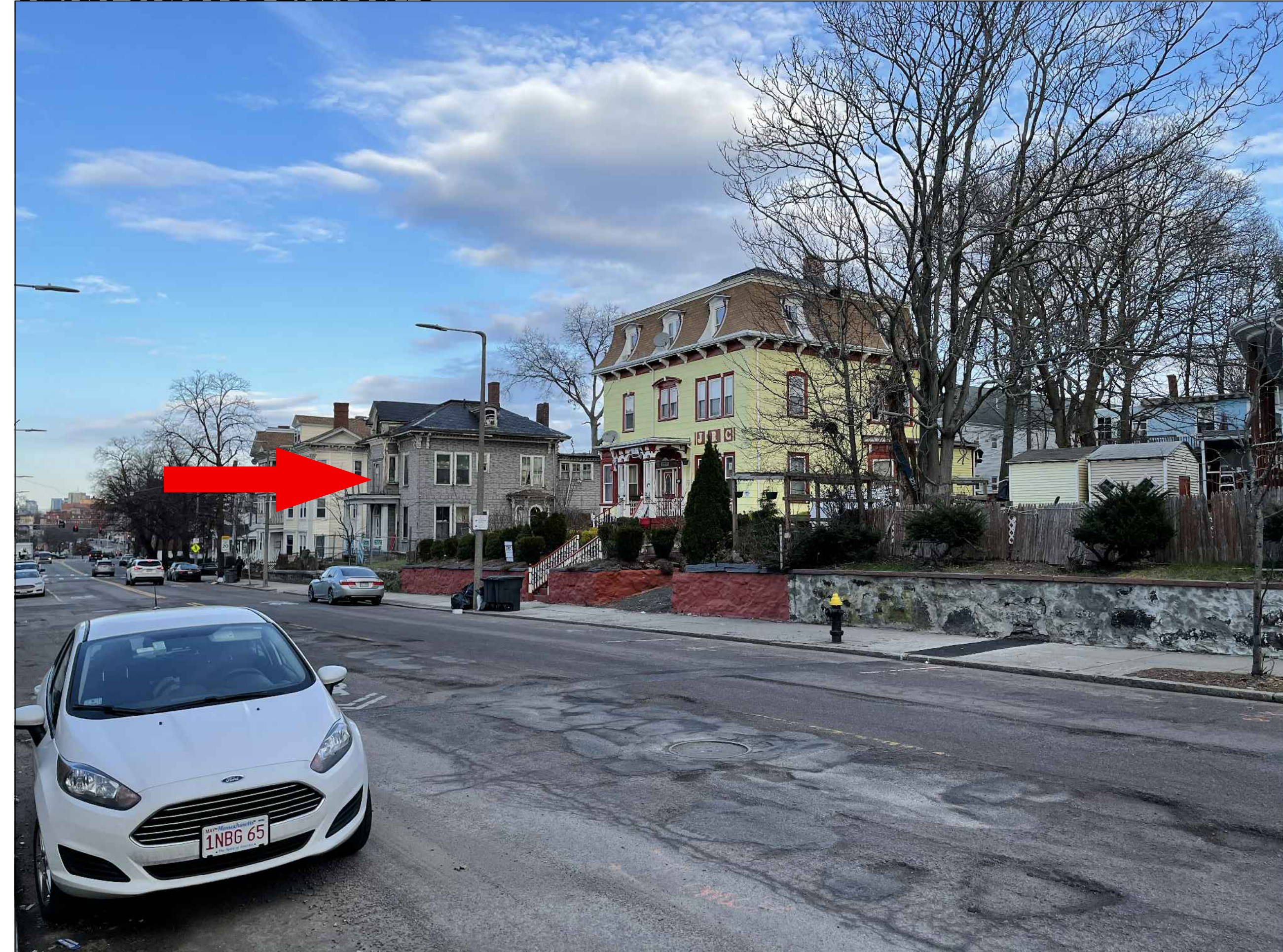
VIEW DOWN WARREN FROM THE SOUTH
