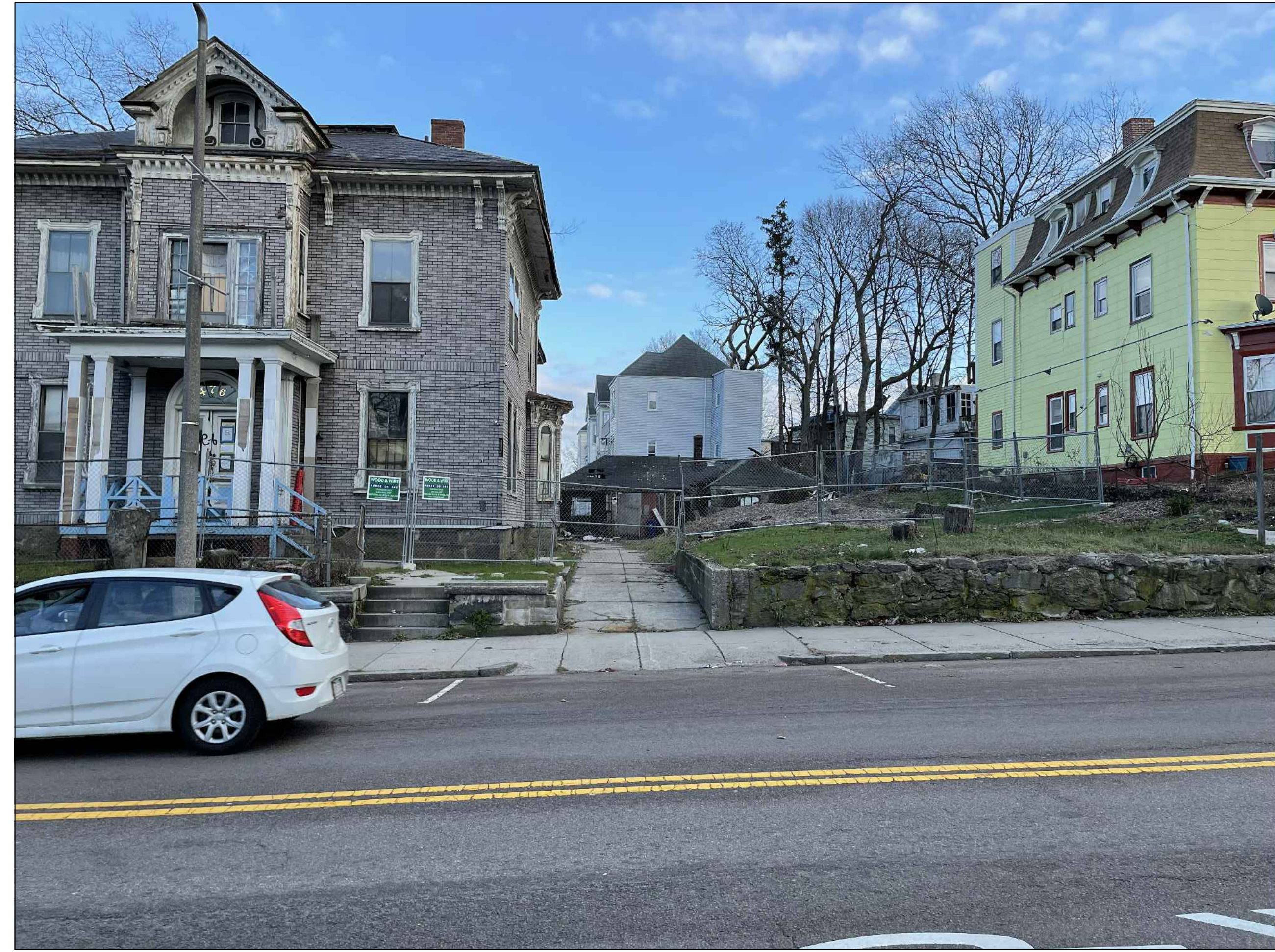
REAR GARAGE EXISTING
