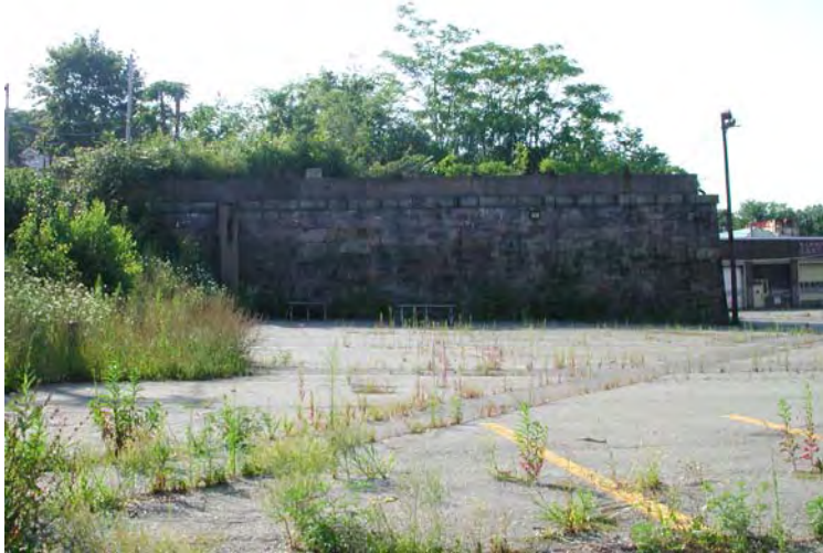
Washington St. at Guild / Retaining Wall
