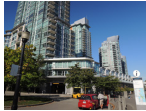
Figure 165. A series of towers are linked by a common podium that is active in use along the main pedestrian thoroughfare, Vancouver, BC.
