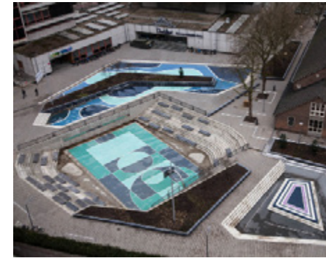
Figure 156. Multi-use detention basin, Rotterdam, Netherlands
