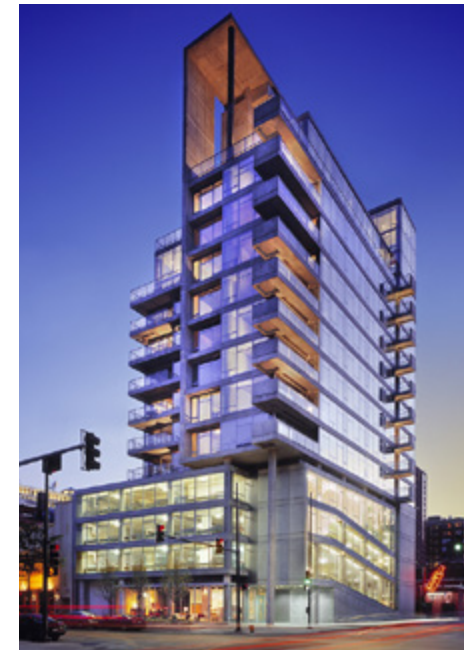
Figure 171. The podium garage is clad in high quality glazing that matches the tower above, Contemporaine, Chicago.
