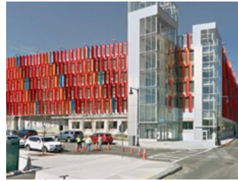
Figure 168. The garage is screened with a creative, bright pattern that adds to the character of the district. Murals are another placemaking strategy for garages, New Balance Headquarters, Boston
