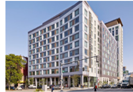
Figure 170. The structured parking is wrapped with residences and an active ground floor, Troy Apartments, Boston
