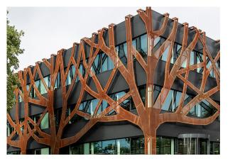
Garage reference — laser cut screen concealing parking decks
