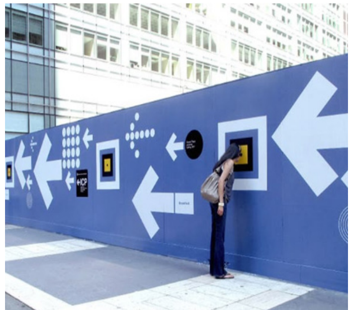
Example of a construction edge that integrates educational elements and clear wayfinding to guide movement around active work zones.
