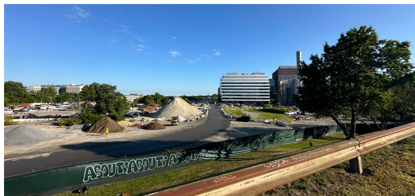
Existing view from Trotting Avenue looking north.
