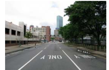
3 HERALD – ACCESS STREET
