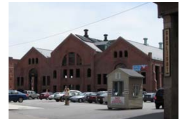
4 FORMER POWER STATION
