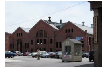
3 FORMER POWER STATION
