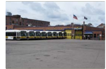
4 MBTA BUS GARAGE
