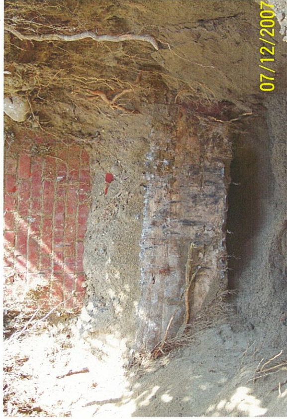
Test Pit JE-TP2 Exposed Foundation and Exposed Bottom of Foundation Rear of Building
