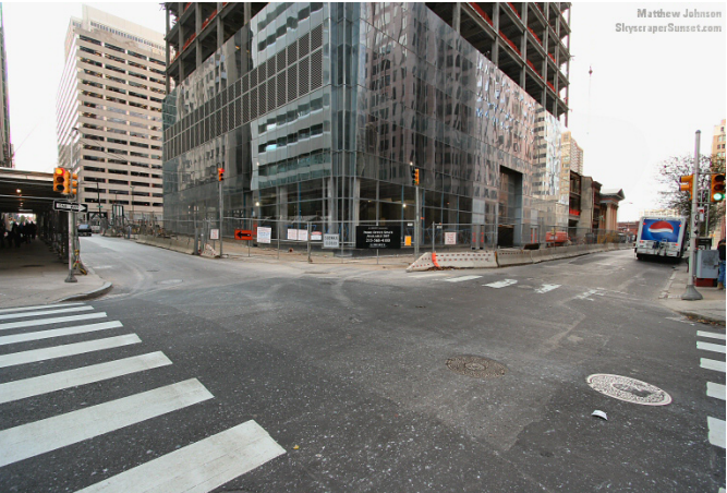
The Comcast Building in Downtown Philadelphia completed the glass façade around the building while they were still building the upper layers. This provided a cleaner and more interesting construction site (there is no opaque hoarding; rather, the area remains open for the public to view the progress). In addition, they continued the glass cladding as building progressed thereby providing viewer interest.
