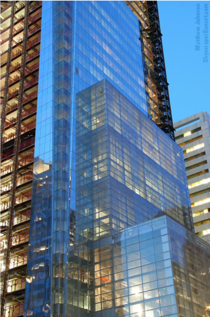
The Comcast Building in Downtown Philadelphia completed the glass façade around the building while they were still building the upper layers. This provided a cleaner and more interesting construction site (there is no opaque hoarding; rather, the area remains open for the public to view the progress). In addition, they continued the glass cladding as building progressed thereby providing viewer interest.
