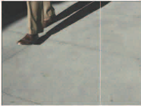
Figure 3.4b An example of smooth, finished concrete sidewalk with saw-cut joints and a dark, fine surface aggregate in downtown Boston
