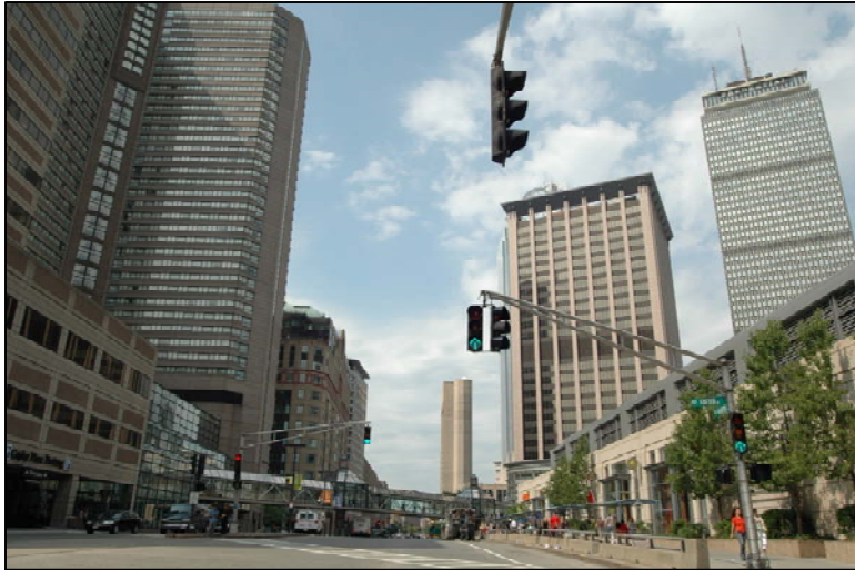
View Southwest from Huntington Avenue of the Project site (left) and the Prudential Center (right)
