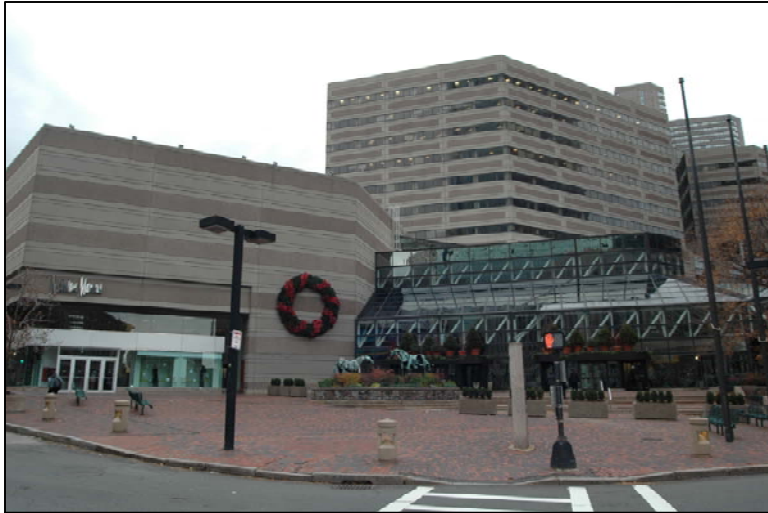
View Southwest from the intersection of Stuart Street and Dartmouth Street to the Project site
