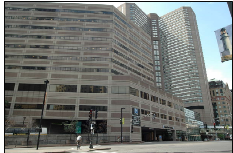
View Southwest to the Project site from the Corner of Avenue of the Arts and Stuart Street
