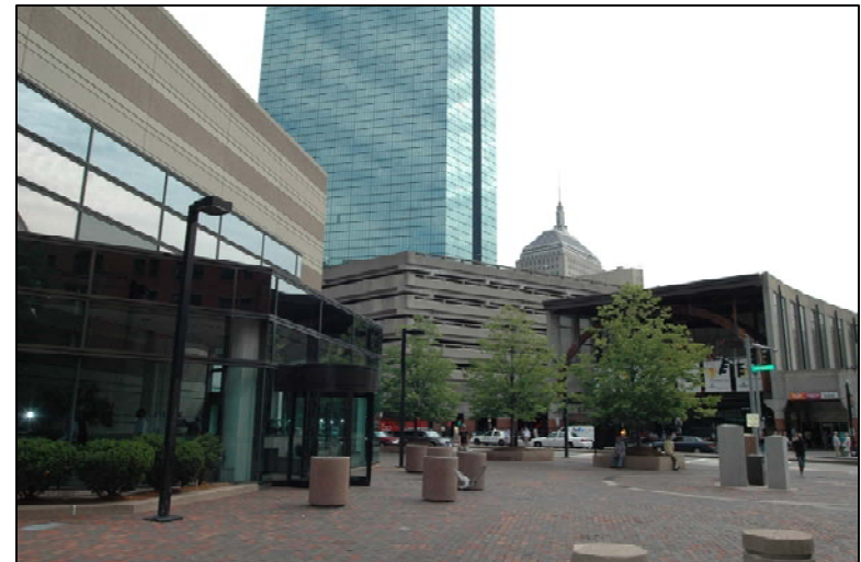
View Northeast to the Project site and MBTA Back Bay Station from the Southwest Corridor Park
