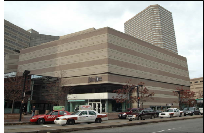
View West to the Project site and the Southwest Corridor Park from Dartmouth Street
