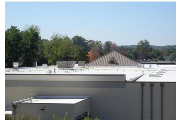
Boston's Seaport Hotel employs an extensive green roof with hardy grasses and sedums to reduce roof stormwater runoff and the heat island effect (top). A high albedo, white TPO membrane (bottom) reflects heat from a supermarket to reduce the need for building cooling and use less energy, as well as to lessen local heat island effects.
