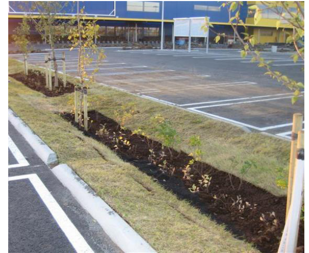
Natural infiltration of stormwater is facilitated by bioswales, such as these at a retail store parking lot.
