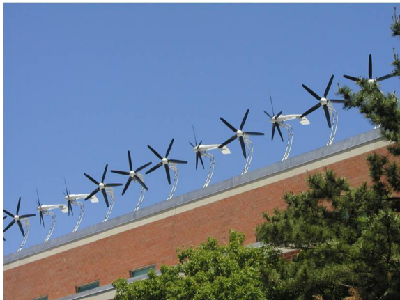
Ceiling skylights in a supermarket provide natural, energy-efficient daylighting (top). Roof-mounted micro-turbines enable harnessing of wind energy in an urban environment, as demonstrated by Massport's project at Boston Logan International Airport (bottom).
