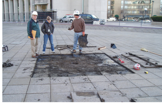
2. Working on the Reflecting Pool membrane.
