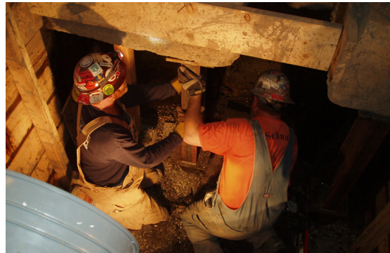
3. Working on wood piles beneath the Church edifices.
