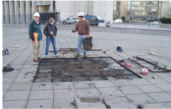
2. Working on the Reflecting Pool membrane.
