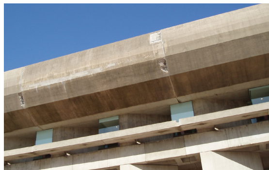
5. Example of deteriorating facades on the Plaza buildings.
