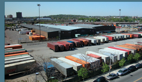
Allston Landing North
