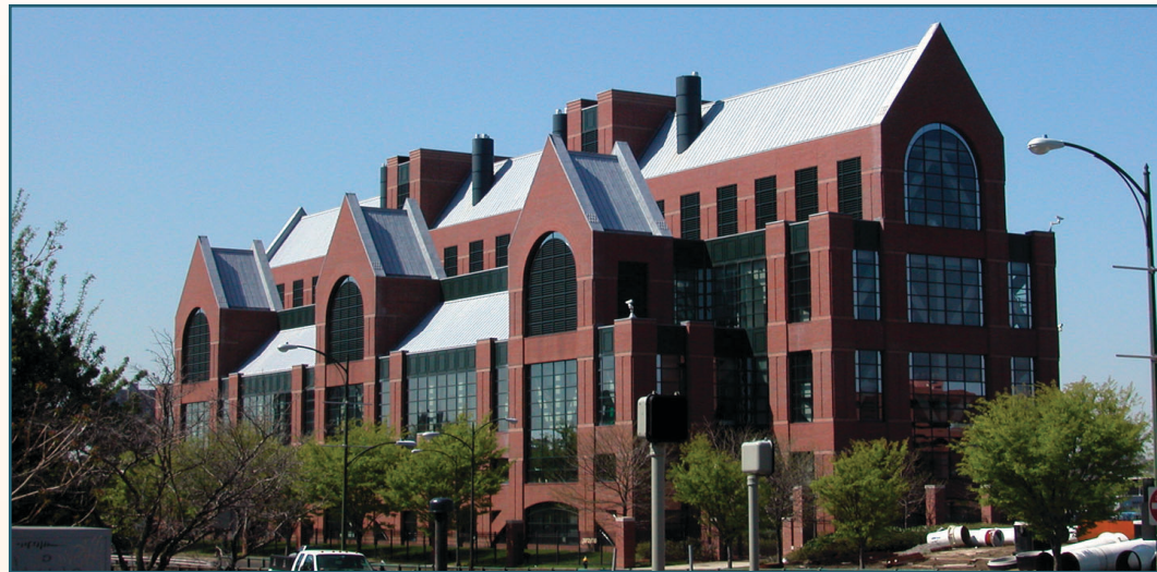
Biotech leader Genzyme's manufacturing facility in North Allston represents new economic vitality for the community, the City, and the region.
