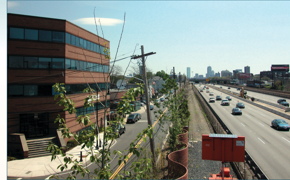
Cabot, Cabot and Forbes demonstration noise-reduction wall is an example of private investment in North Allston's public amenities.
