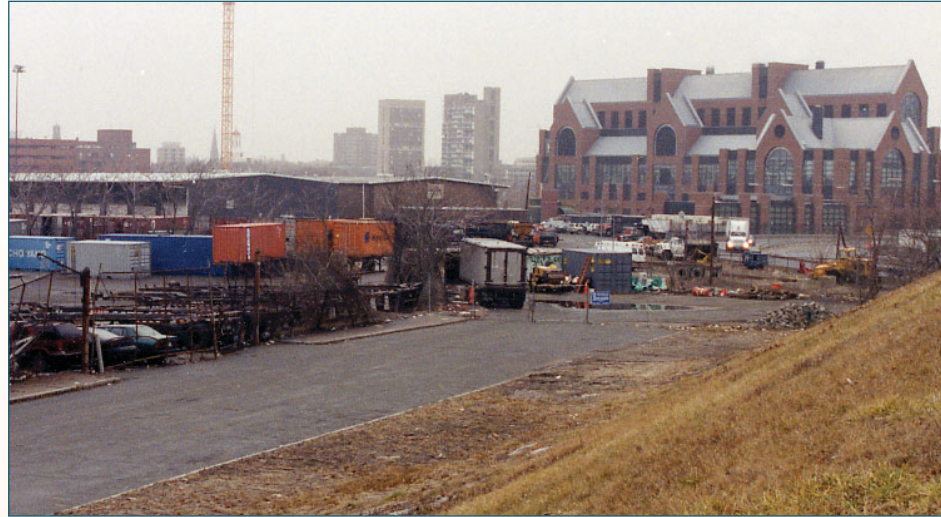
The transportation assets located in Allston Landing North, seen here looking toward the Genzyme manufacturing facility along Soldiers Field Road, contribute to the major resources for maintaining the economic health of the area and the region.
