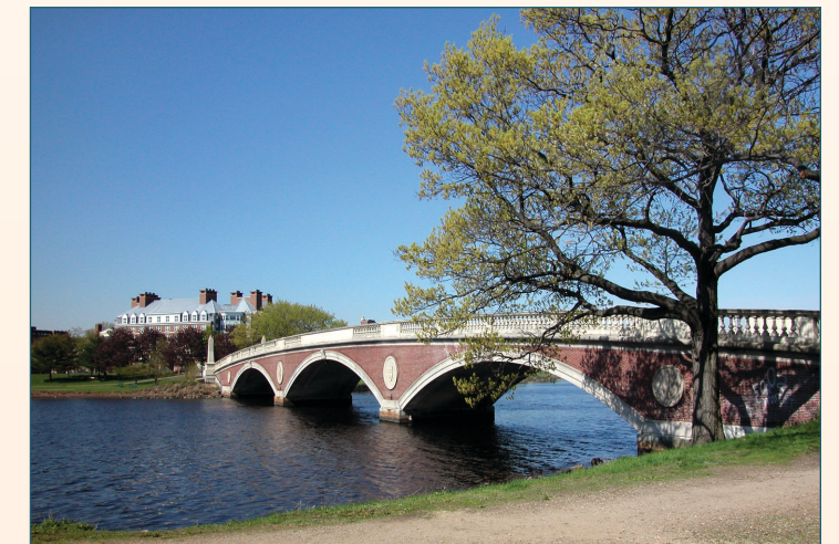
The Weeks Bridge serves as a pedestrian connection between Harvard's Cambridge and North Allston campuses.
