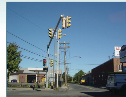
Existing conditions: Looking north on Everett Street.
