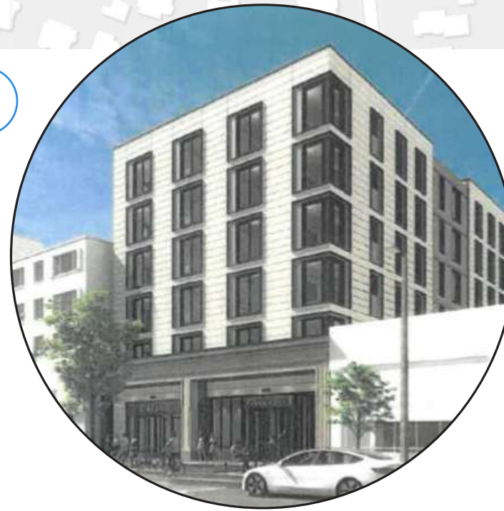
1035 Comm Ave (Under Construction)
