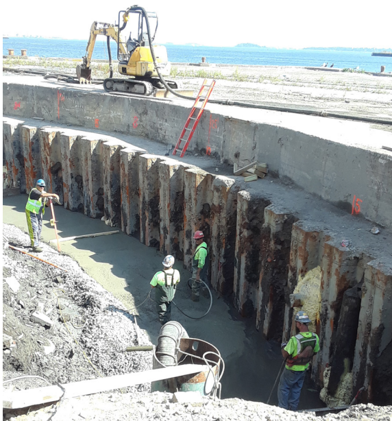
East Jetty Construction
