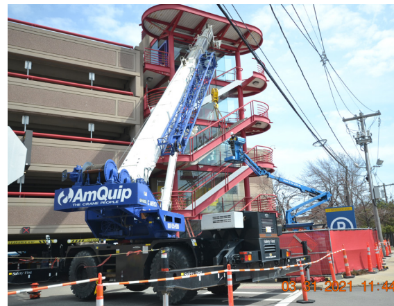
Marine Park Garage Construction
